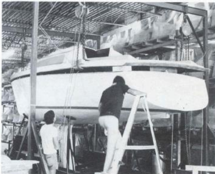
The prototype gets its trial cabin top at BYRD, Summer 1982. (In the background are railway seats using the closed mould process.)
